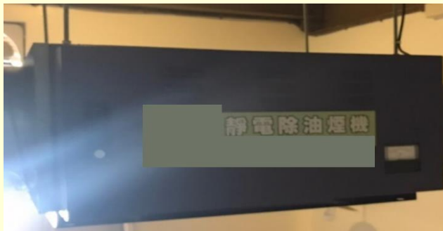
(油煙防制設備)
