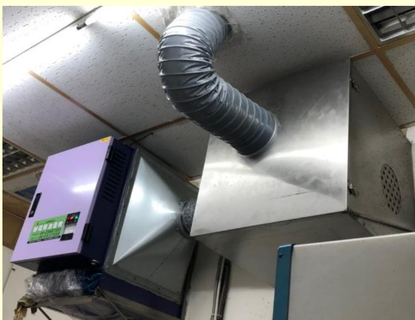
(油煙防制設備)
